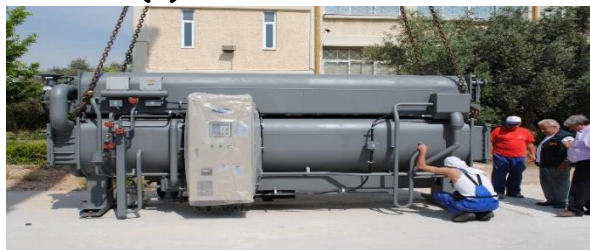
Fig. 8. The general view of the plant (a), the power couple (b) and the absorption chiller (c)
